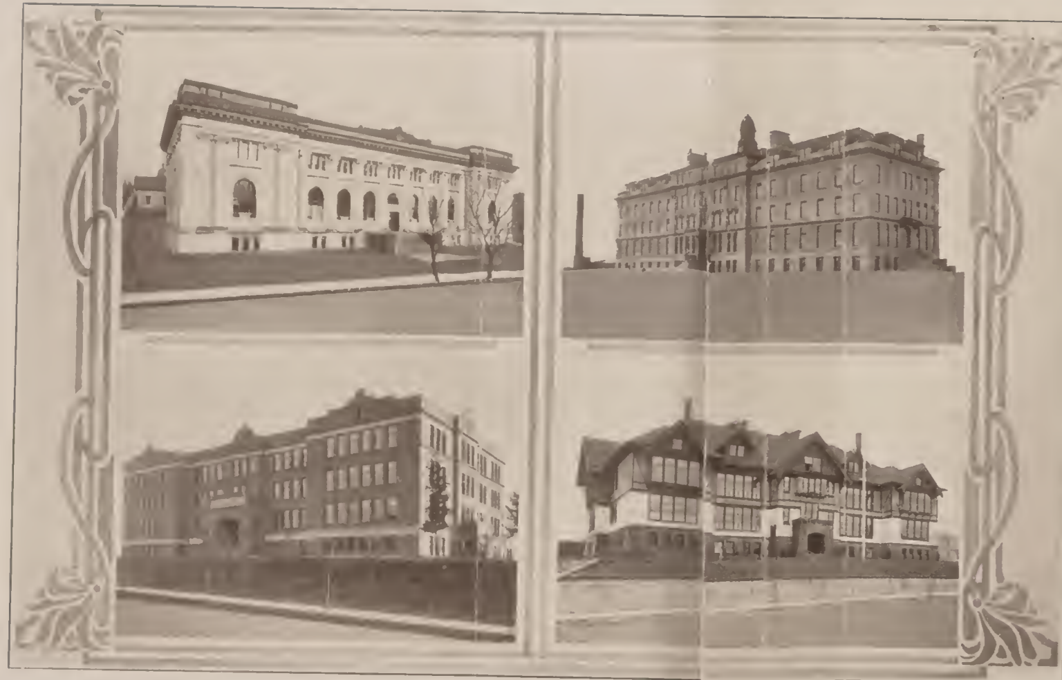
A FEW OF THE MANY PUBLIC BUILDINGS OF THE CITY. (1) Public Library. (2) House of Good Shepherds. (3) Lincoln High School. (4) Franklin School.
